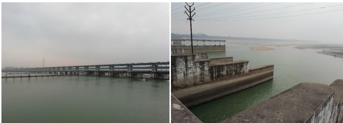
Figure 8: Gandak Barrage showing the water depth difference in Nepal (left) and India (right) side
